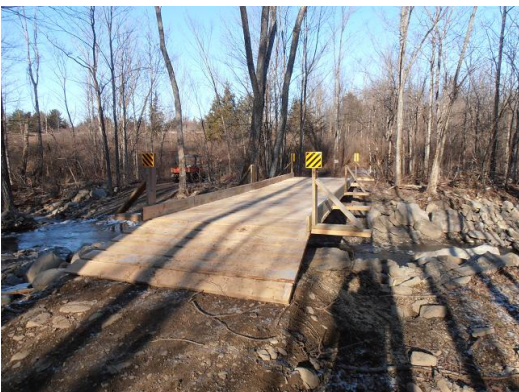
On left, the Esperance Auto bridge restored higher than before.
