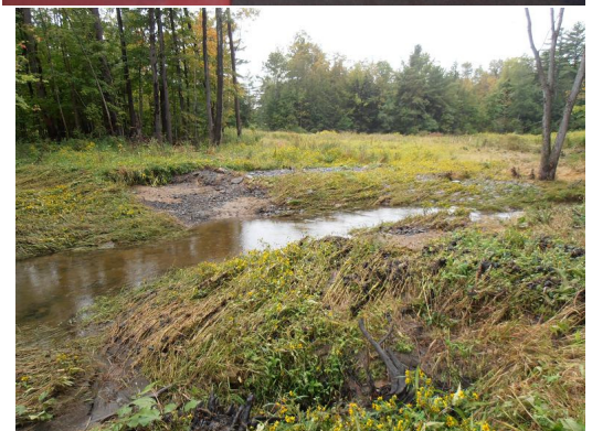
On right, days after Irene washed away the long Rt146 bridge. We've come a long way from that day.
